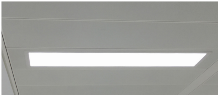
Flatline 1200 x 300mm, within a tile - 25 Knightsbridge Installation
