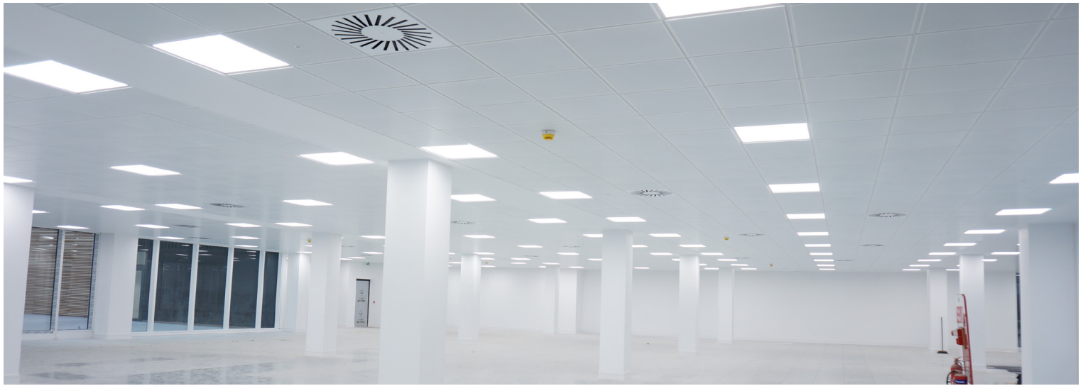
FLATLINE installation at Westside, Hemel Hempstead.
