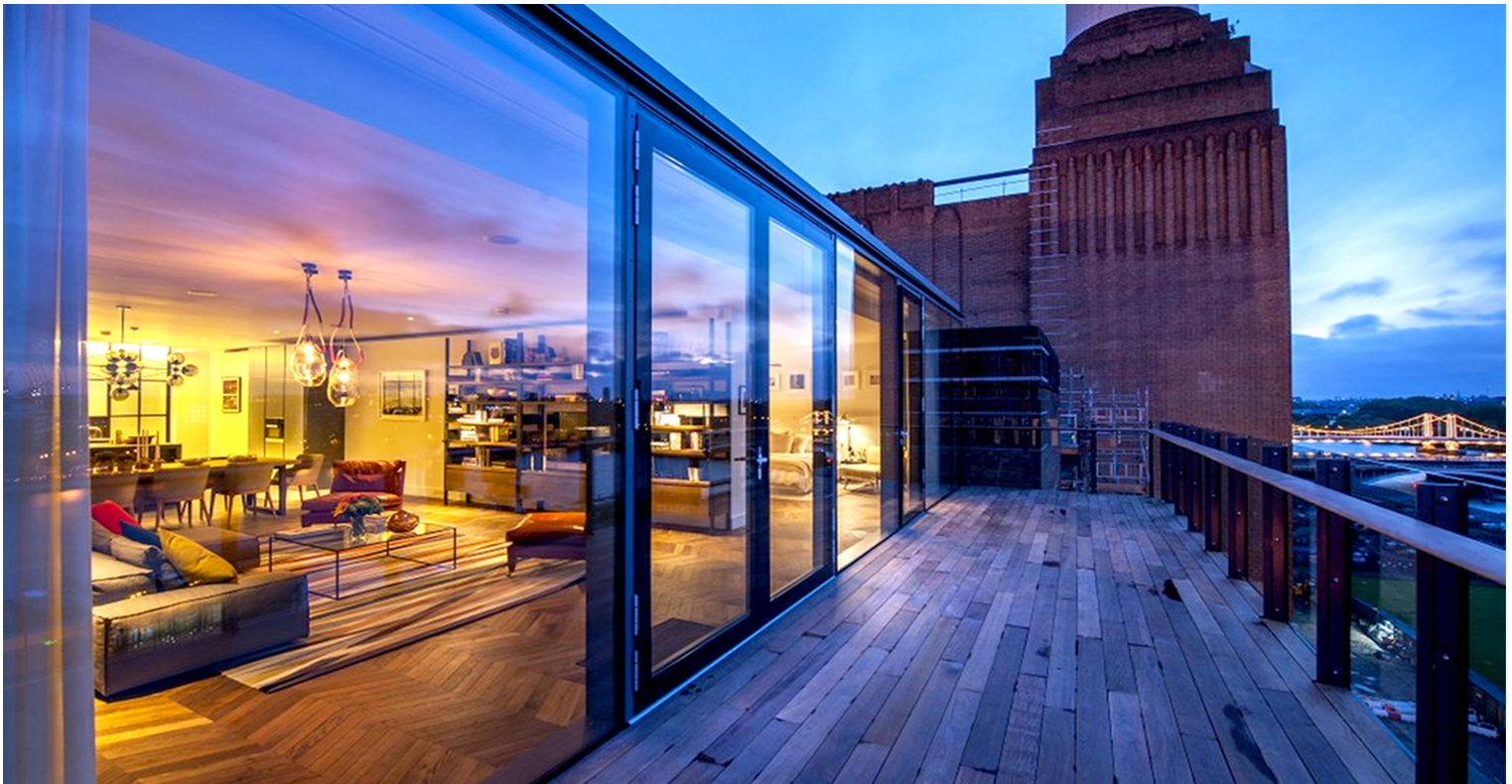
Battersea Power Station - Over 25,000 ILS Fittings supplied
